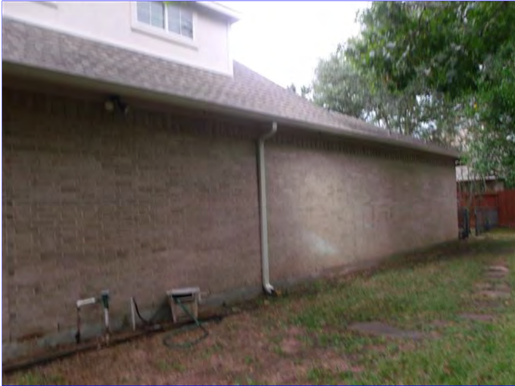
B. Item 4(Picture) Downspouts should drain water a minimum five feet away from the foundation.
