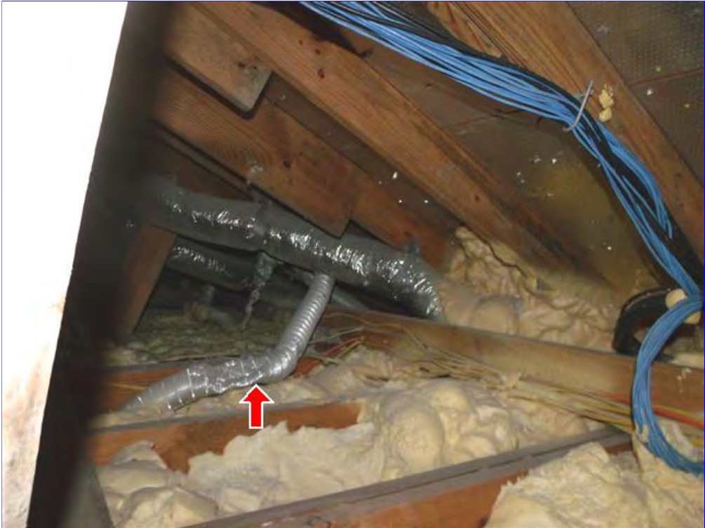
G. Item 1(Picture) Bathroom exhaust is crushed and it venting into the attic. In need of repair.
