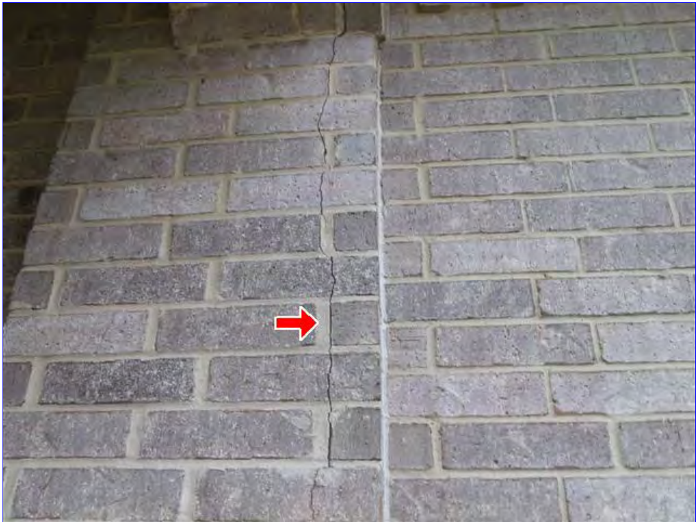
D. Item 13(Picture) Crack under the archway.
