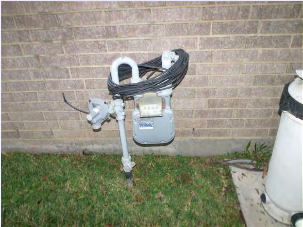
E. Item 2(Picture) Gas meter should be bonded and grounded.
