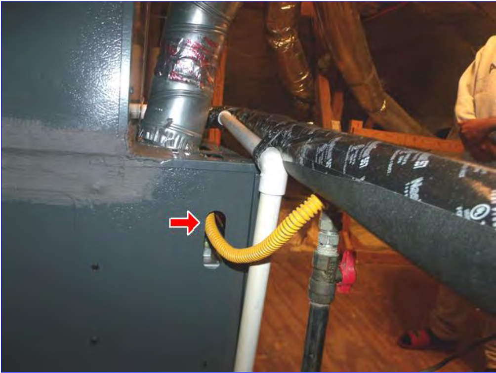
B. Item 4(Picture) Improper connection. In need of repair.
