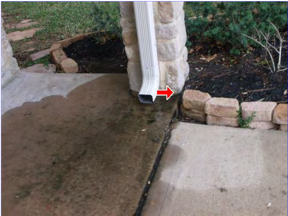
B. Item 2(Picture) Sugest turning the downspout away
