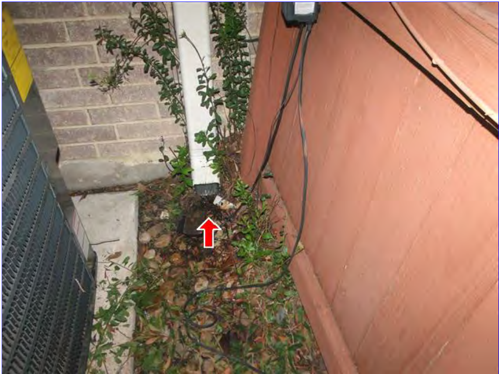
B. Item 13(Picture) Downspout should discharge away from the foundation and electrical equipment.
