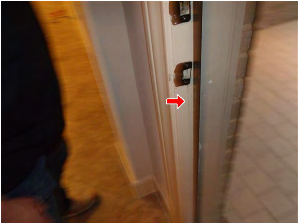
F. Item 1(Picture) Damaged latch. Recommend repair.
