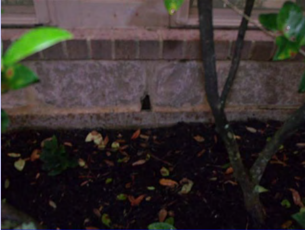
A. Item 7(Picture) Should have a minimum of four inches of exposed slab for masonry.
