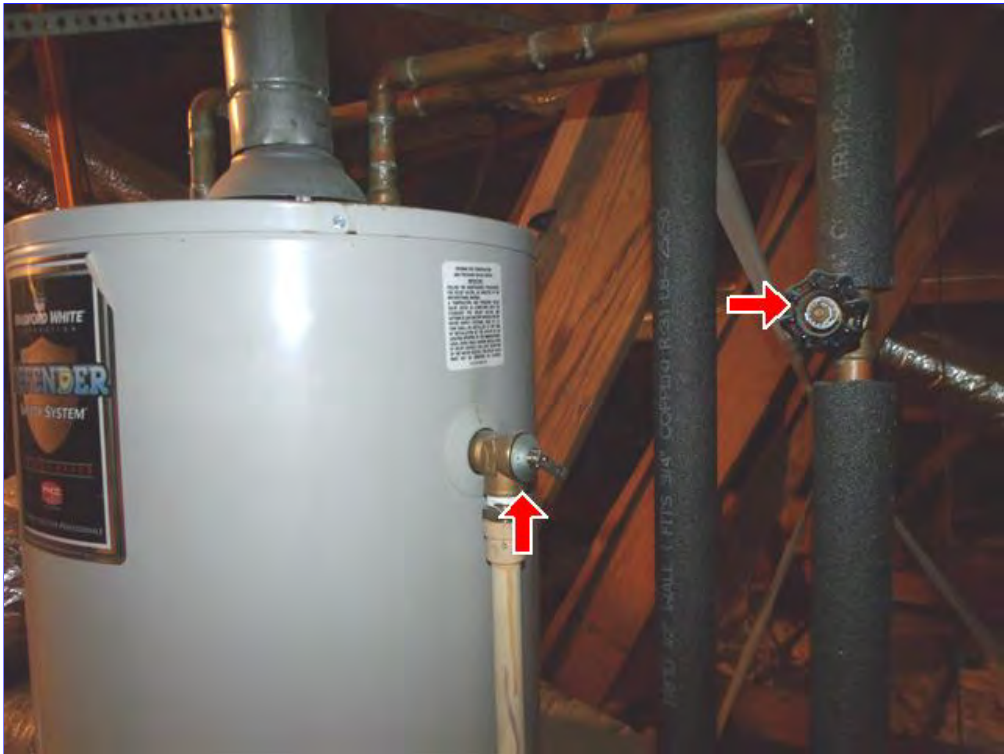
C. Item 3(Picture) T&PV was in good condition at the time of inspection. Cold water shutoff valve correctly installed.
