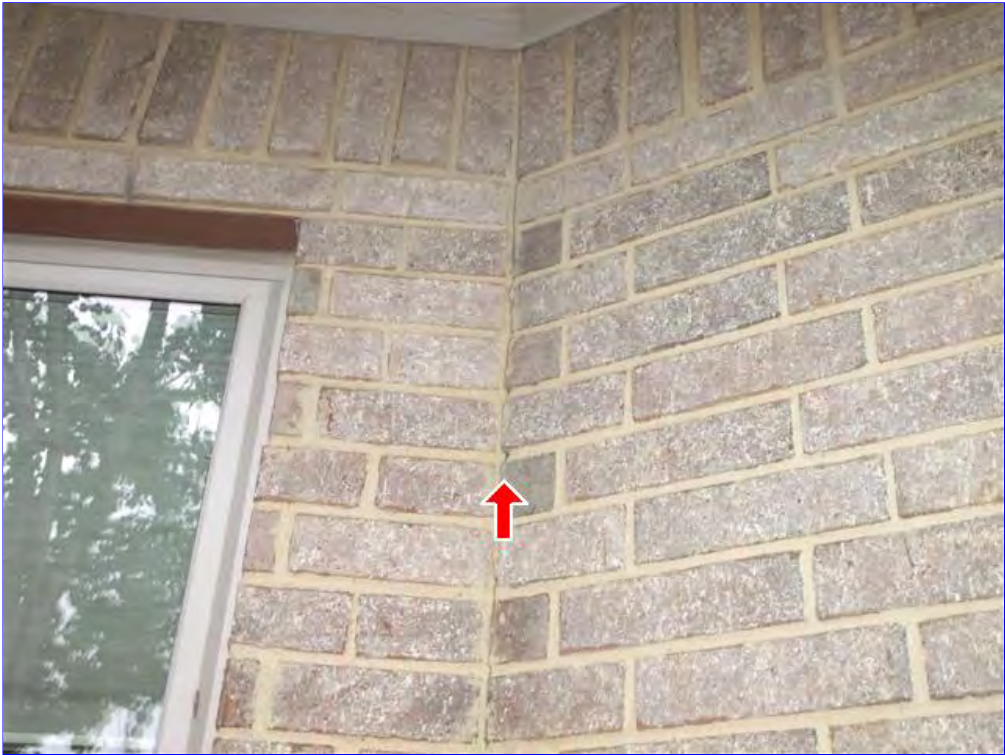
D. Item 10(Picture) Crack in the brick veneer.
