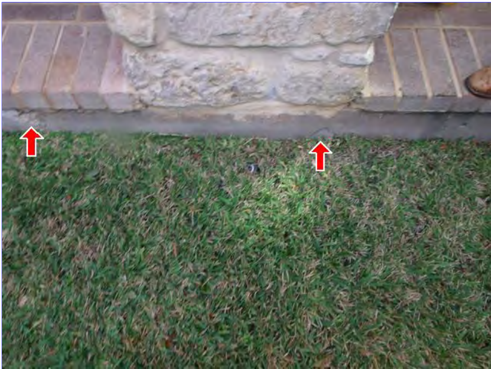
A. Item 16(Picture) Concrete spalling. Recommend sealing with epoxy to prevent water intrusion.
