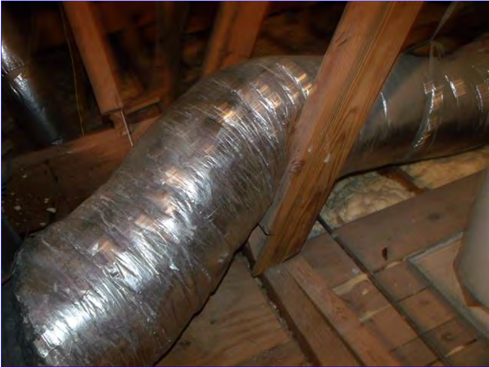
C. Item 22(Picture) Ducts need to be properly strapped.
