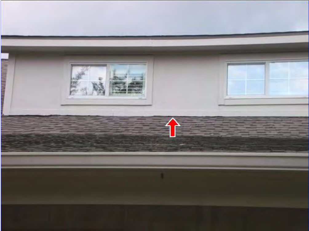
C. Item 1(Picture) Should have a one inch gap between the siding and roofing material.
