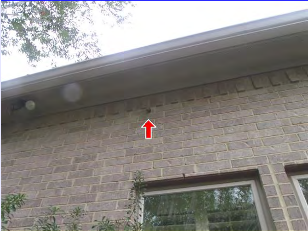
A. Item 13(Picture) Secondary drain located on the left side of the house.
