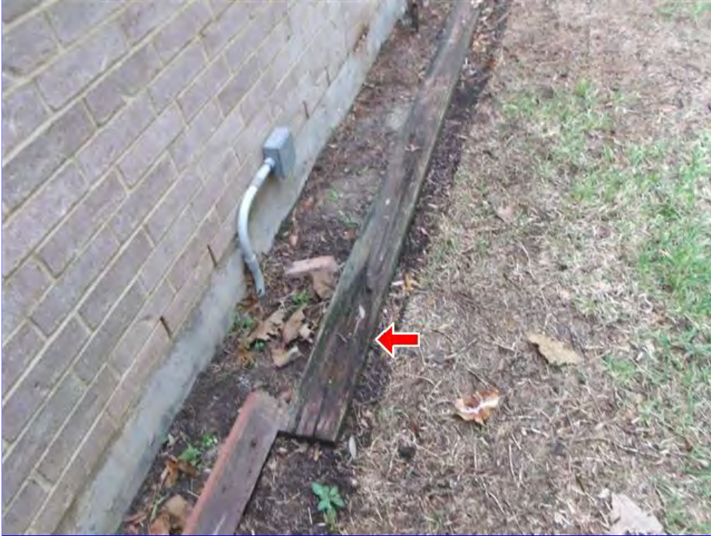
A. Item 9(Picture) Wood is conducive to wood destroying organisms (WDO) and wood destroying insects (WDI).
