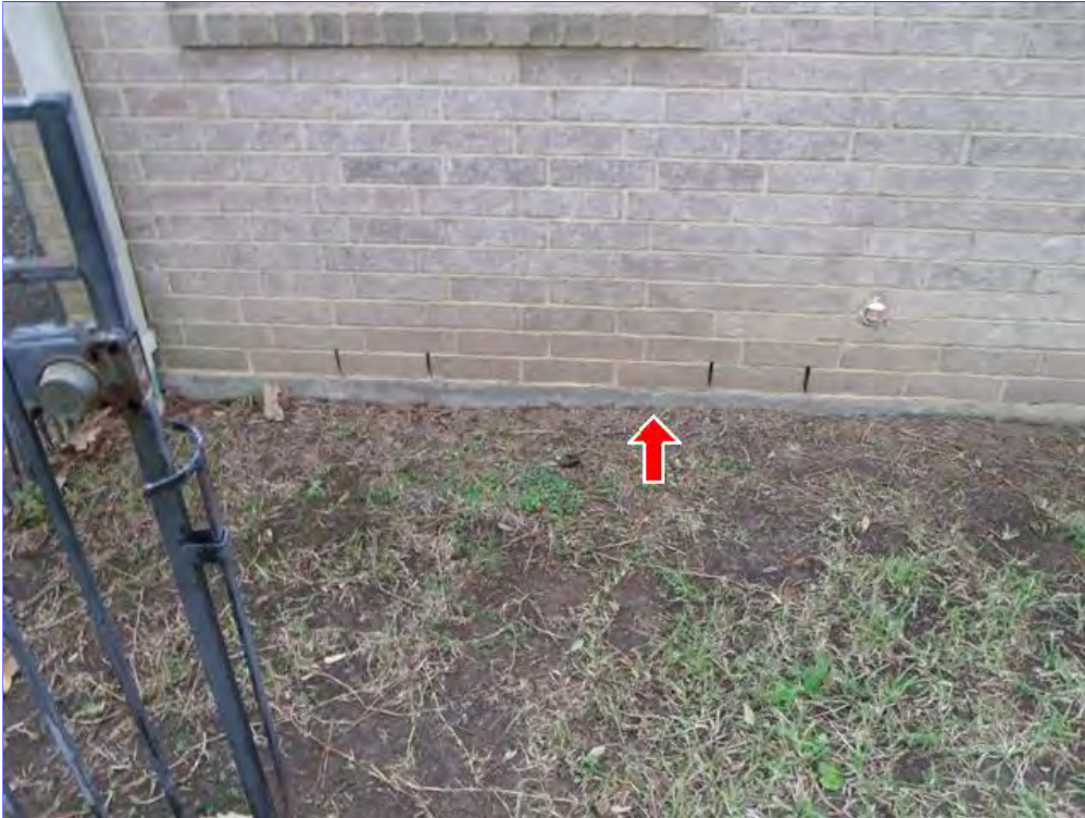
A. Item 10(Picture) Should have a minimum of four inches of exposed slab for brick veneer.
