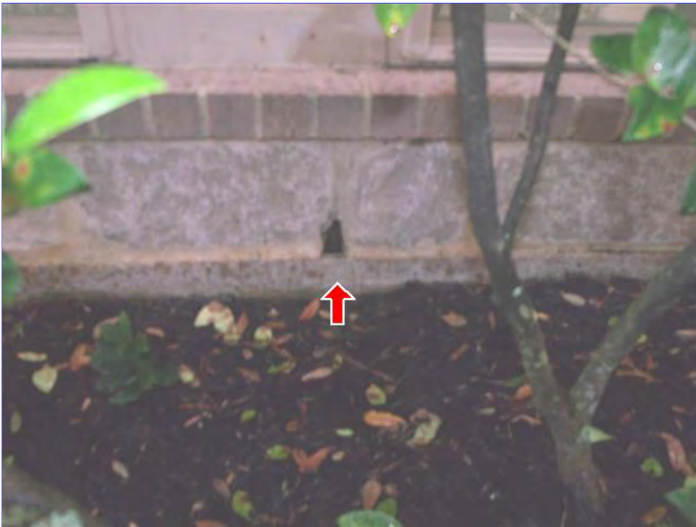
A. Item 4(Picture) Recommend installing weep screens to keep rodents out.
