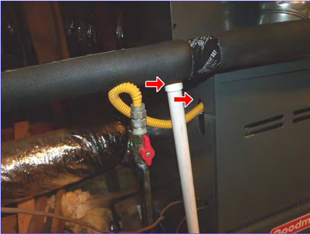
B. Item 10(Picture) Flex line need corrected with solid gas line. Also cap PVC out let line
