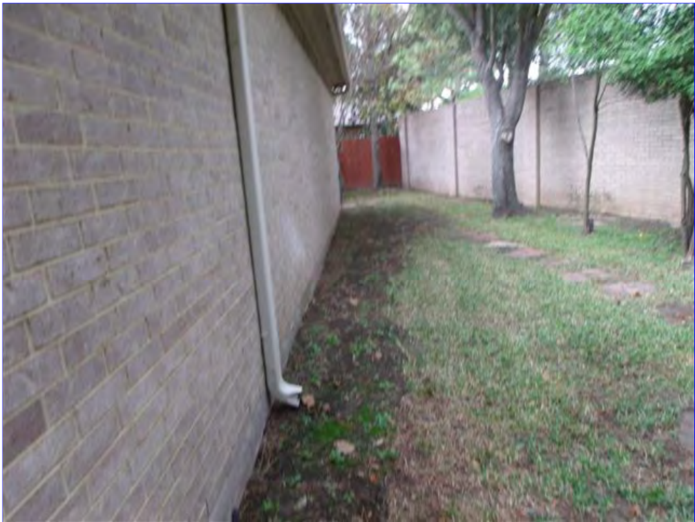
B. Item 8(Picture) Downspouts should drain water a minimum five feet away from the foundation.
