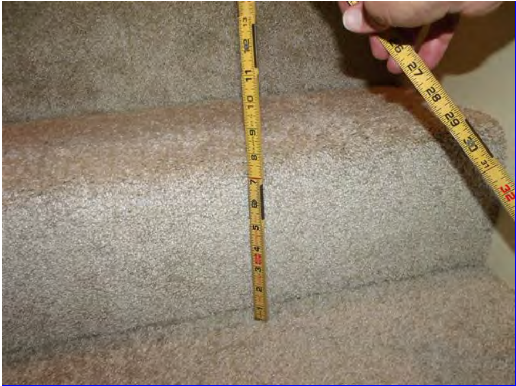
H. Item 6(Picture) Risers are in tolerance.
