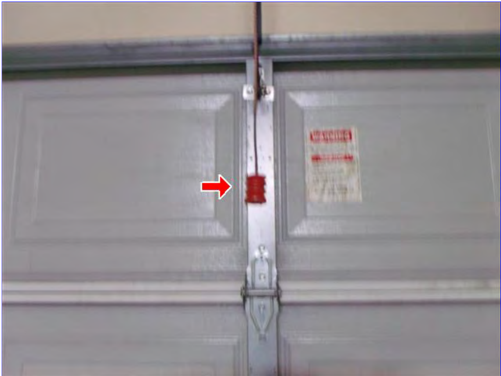
H. Item 3(Picture) Disconnect for the garage door was tested and was operational at the time of inspection.
