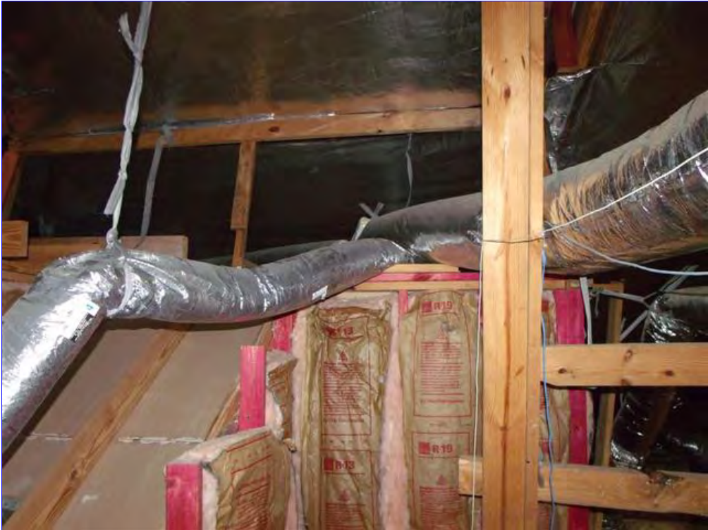
C. Item 3(Picture) Ducts should be strapped every five feet.
