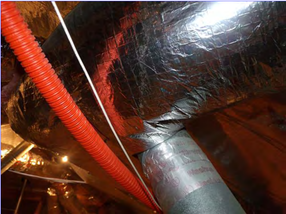
C. Item 21(Picture) Insulation should be installed between the ducts to prevent condensation.
