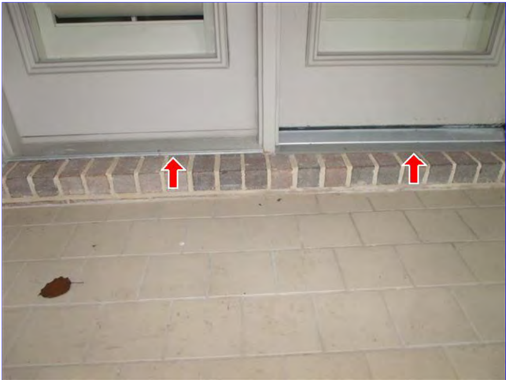
F. Item 2(Picture) Recommend foam caulking underneath thresholds at the backdoors to prevent air intrusion.
