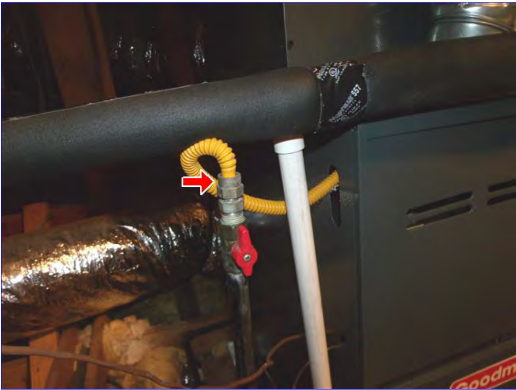
B. Item 2(Picture) Improper connection. In need of repair.
