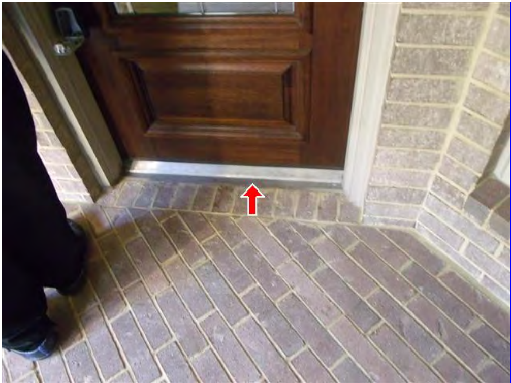
F. Item 3(Picture) Recommend foam caulking underneath thresholds at the frontdoor to prevent air intrusion.
