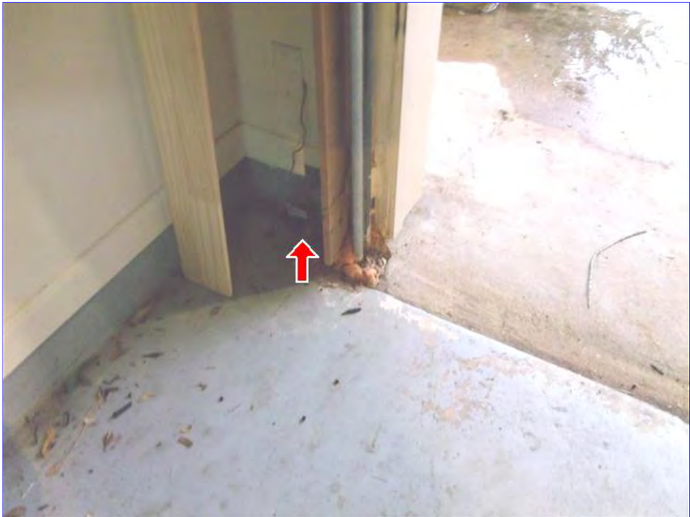
H. Item 1(Picture) Photoelectric sensor needs to be properly secured and be set six inches above the floor. Recommend diverter flashing or screens noted as cloth wire
