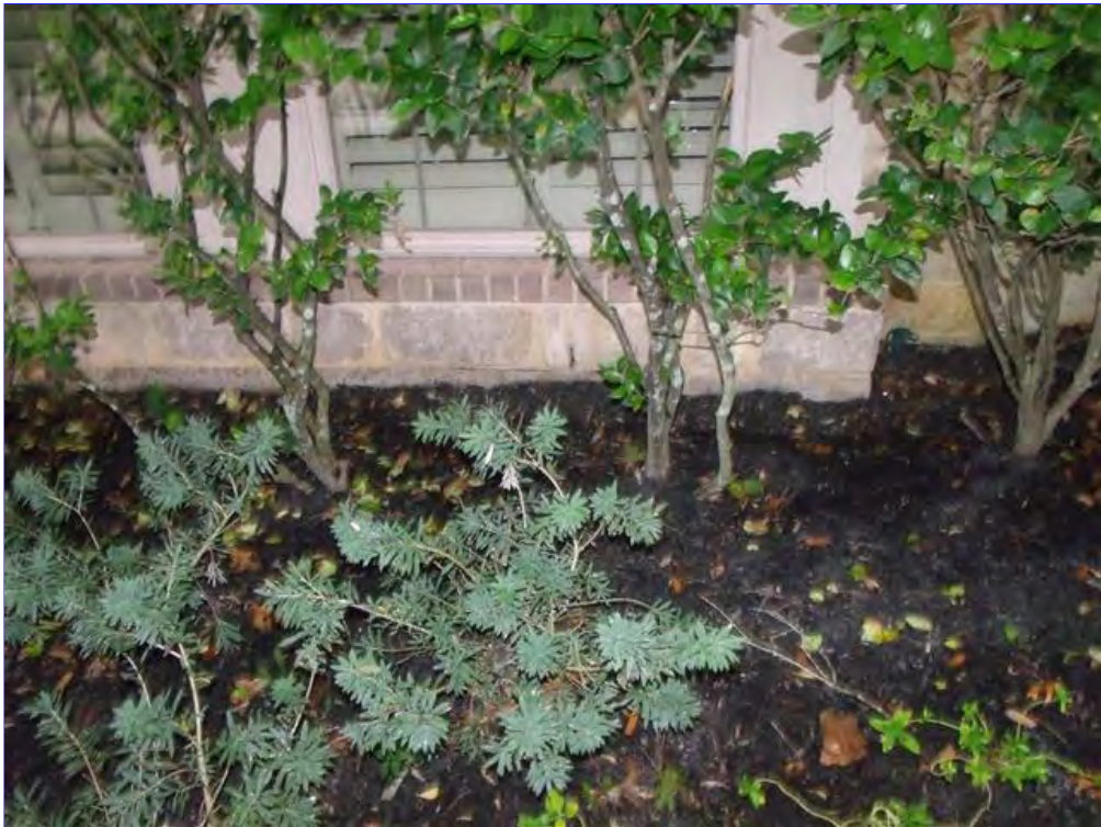
B. Item 3(Picture) Poor grading. Recommend having a six inch slope in ten inches away from the foundation.
