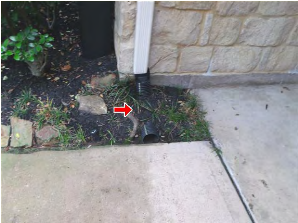
B. Item 5(Picture) Downspouts should drain water a minimum five feet away from the foundation.
