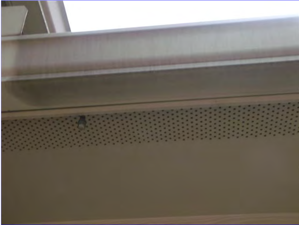
B. Item 6(Picture) Gutter is not discharging water properly.
