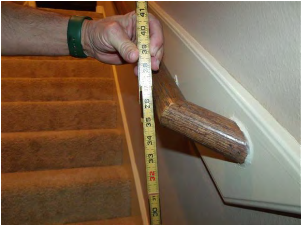
H. Item 3(Picture) Handrail is the proper height.
