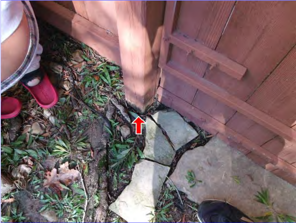
J. Item 1(Picture) Post for the fences are in need of repair.
