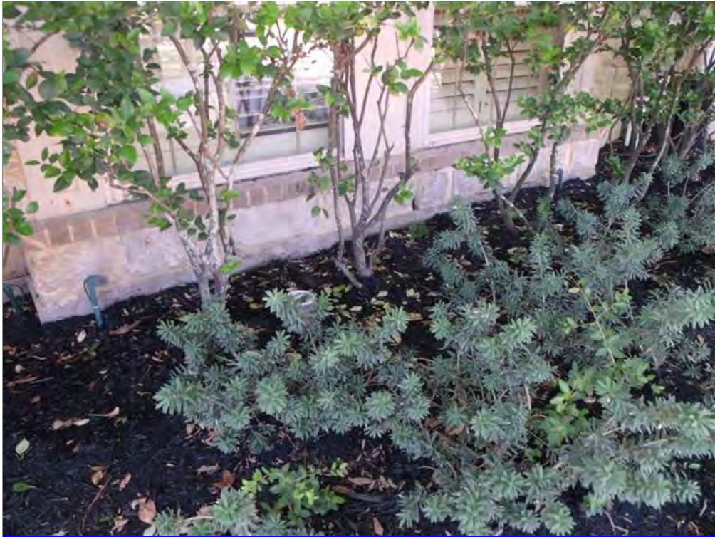
A. Item 18(Picture) It's recommend having four inches of exposed slab. Also proper grading is needed.
