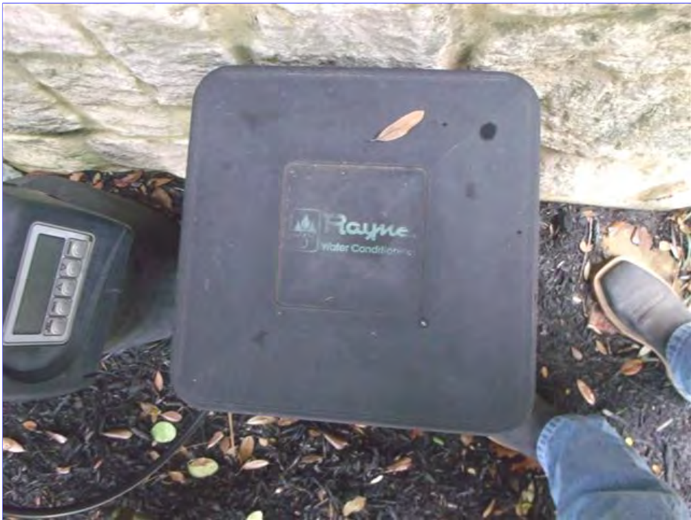
A. Item 6(Picture) Water conditioner for the pond. Its $249.00 for a service call and how to operate unit. Recomend a lockable salt dispenser on unit
