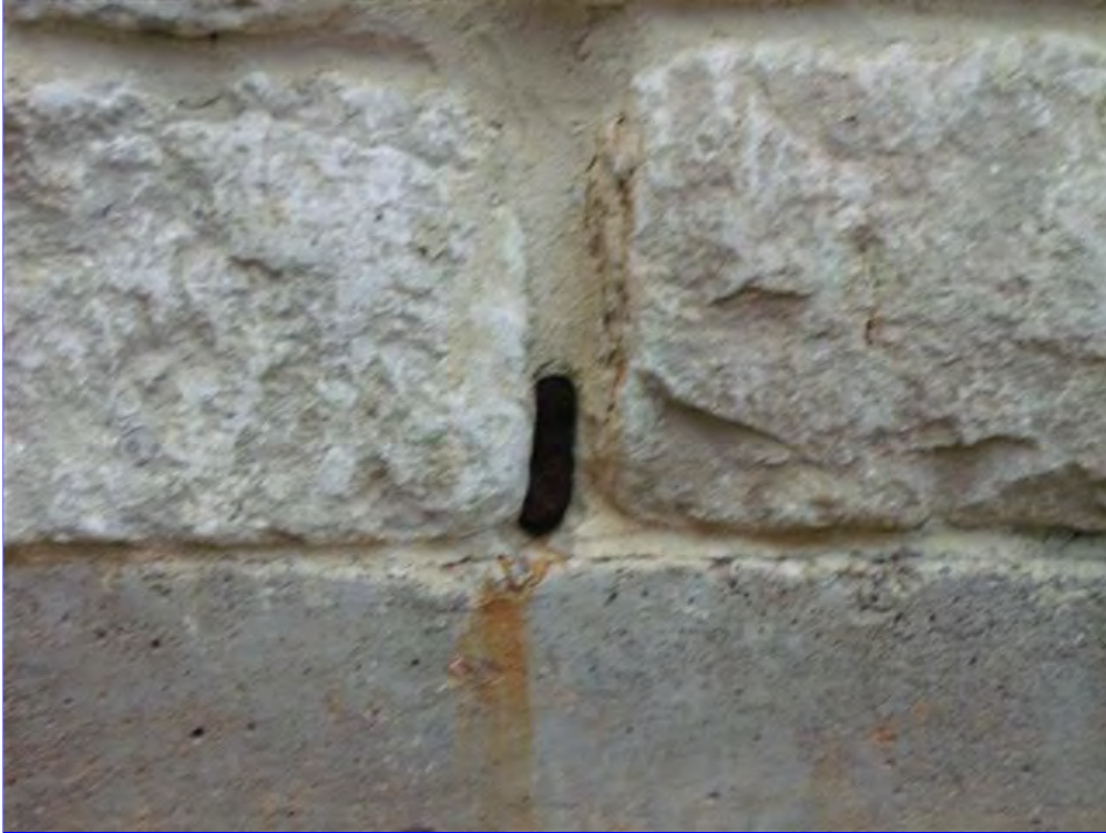
A. Item 5(Picture) Recommend installing weep screens to keep rodents out.
