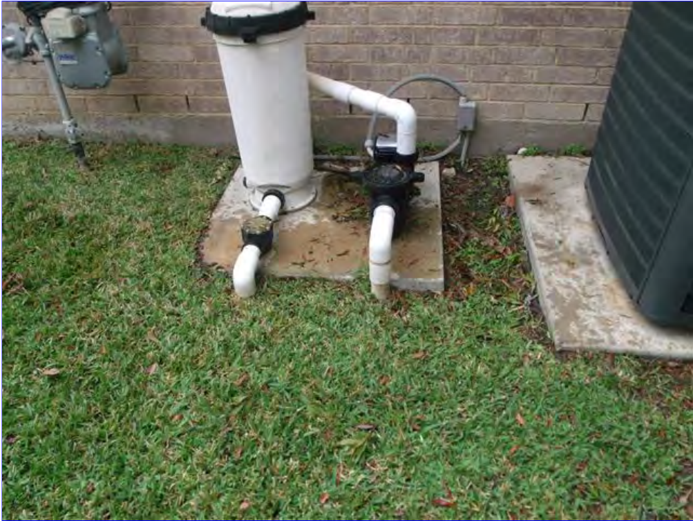
F. Item 1(Picture) Pump needs to be three inches above grade.
