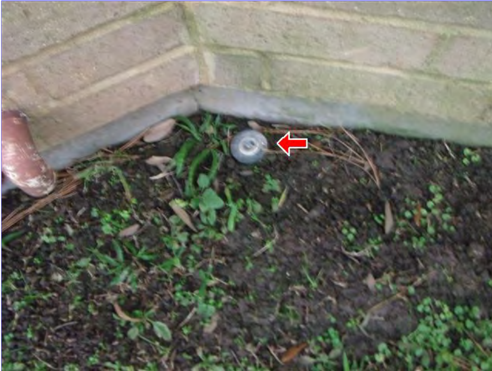
A. Item 14(Picture) Sprinklers too close to the foundation.
