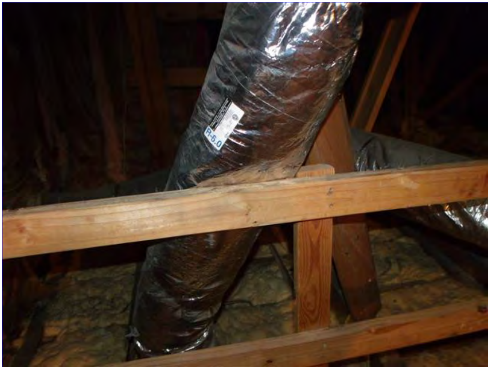
C. Item 2(Picture) Insulation should be installed between the duct and the rail to prevent condensation.
