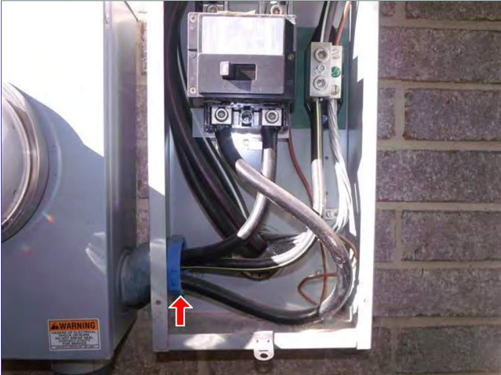
A. Item 8(Picture) Recommend bonding of electrical conduit.
