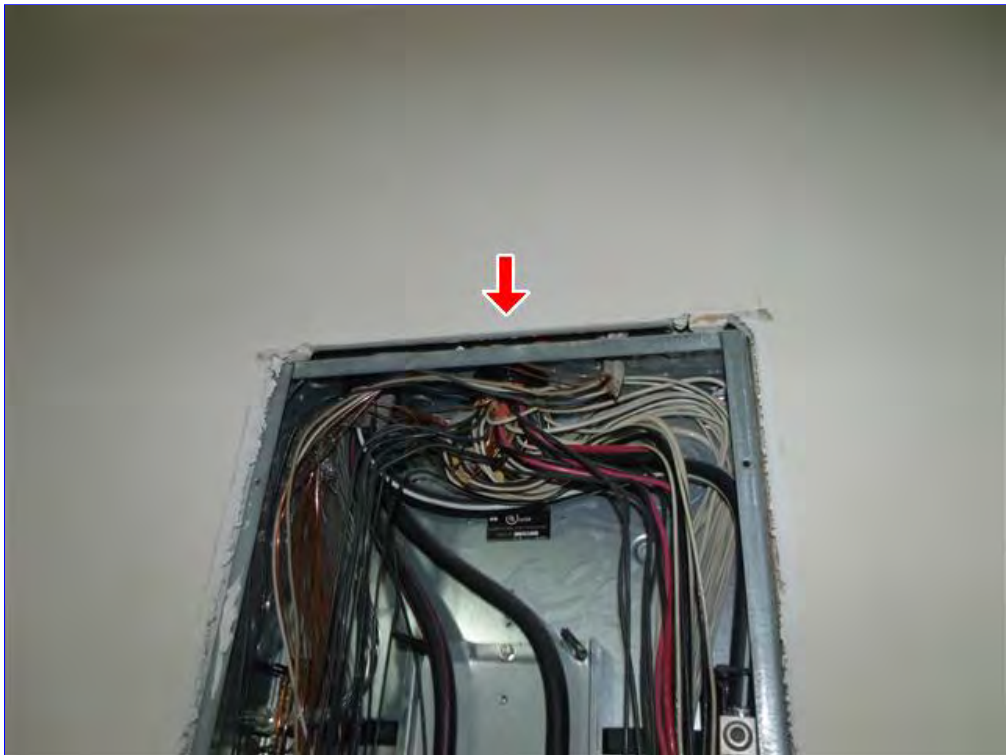
A. Item 4(Picture) Should not have more than one eighth of an inch gap.
