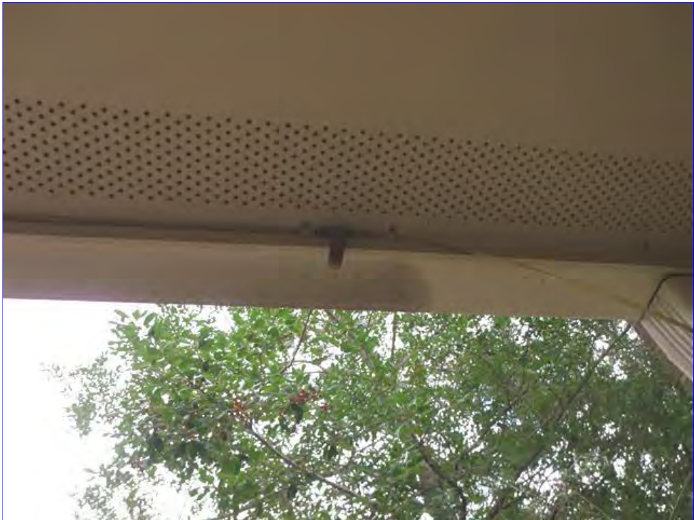
B. Item 7(Picture) Water damage on the fascia.
