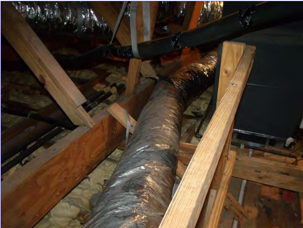
C. Item 23(Picture) Ducts should not be laying on the floor. Recommend strapping every five feet.
