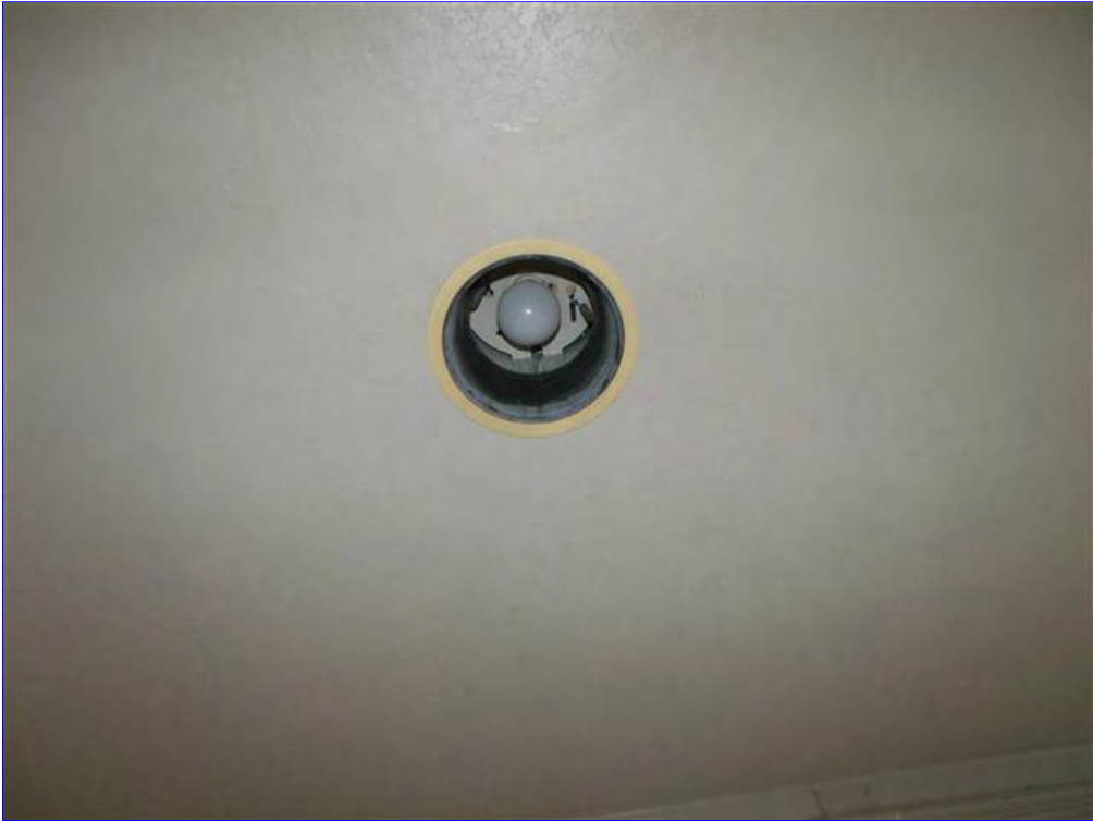
B. Item 6(Picture) Both light fixture need to be installed located under the garage need face plates.
