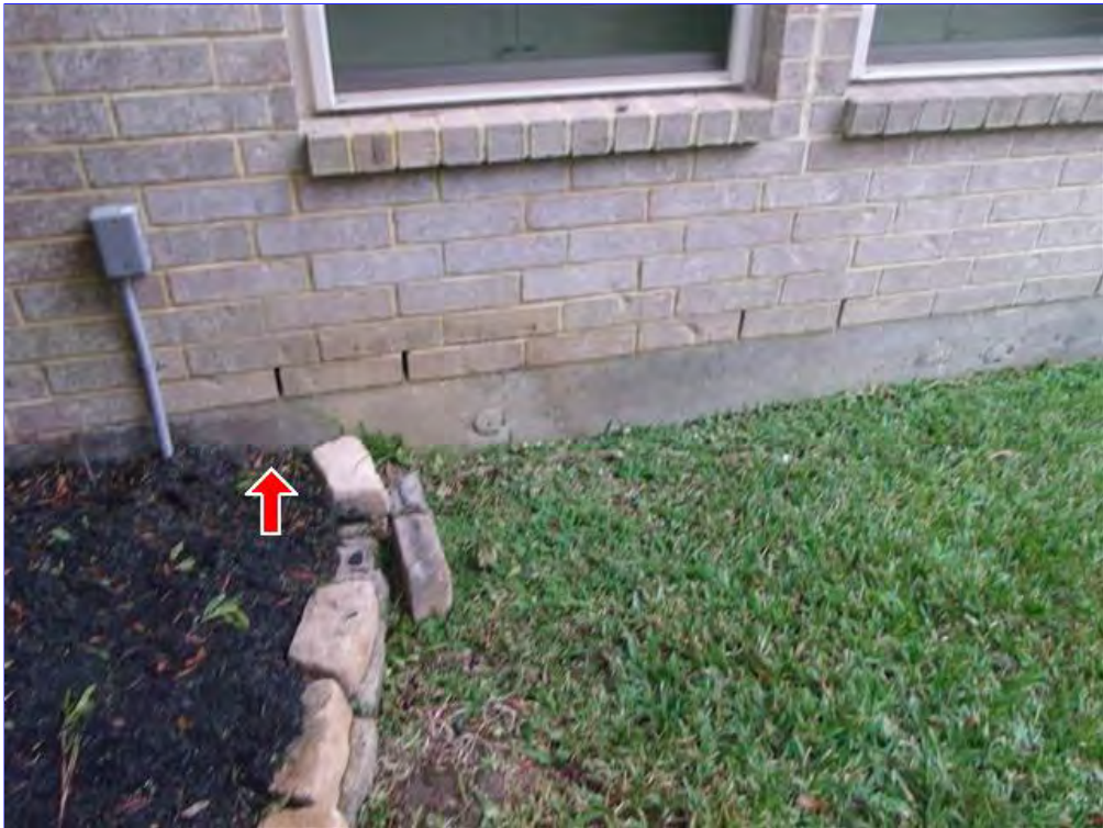
A. Item 15(Picture) Recommend having four inches of exposed slab for brick siding.
