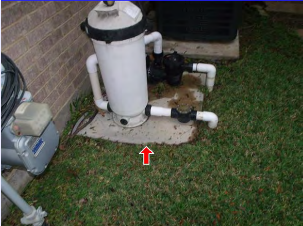
J. Item 1(Picture) Pump needs to be located on a platform at least three inches above grade.
