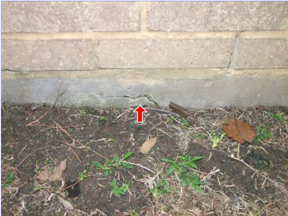
A. Item 17(Picture) Surface crack in the foundation. Recommend sealing with epoxy to prevent water intrusion.
