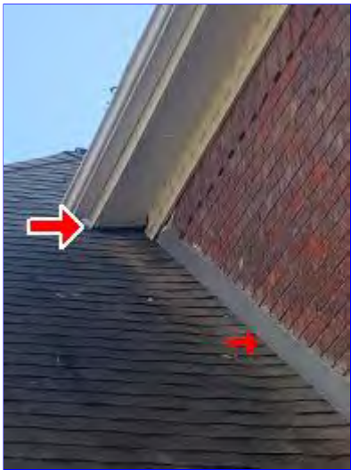
C. Item 10(Picture) This is NOT your roof its a Example of rodent flashing.
