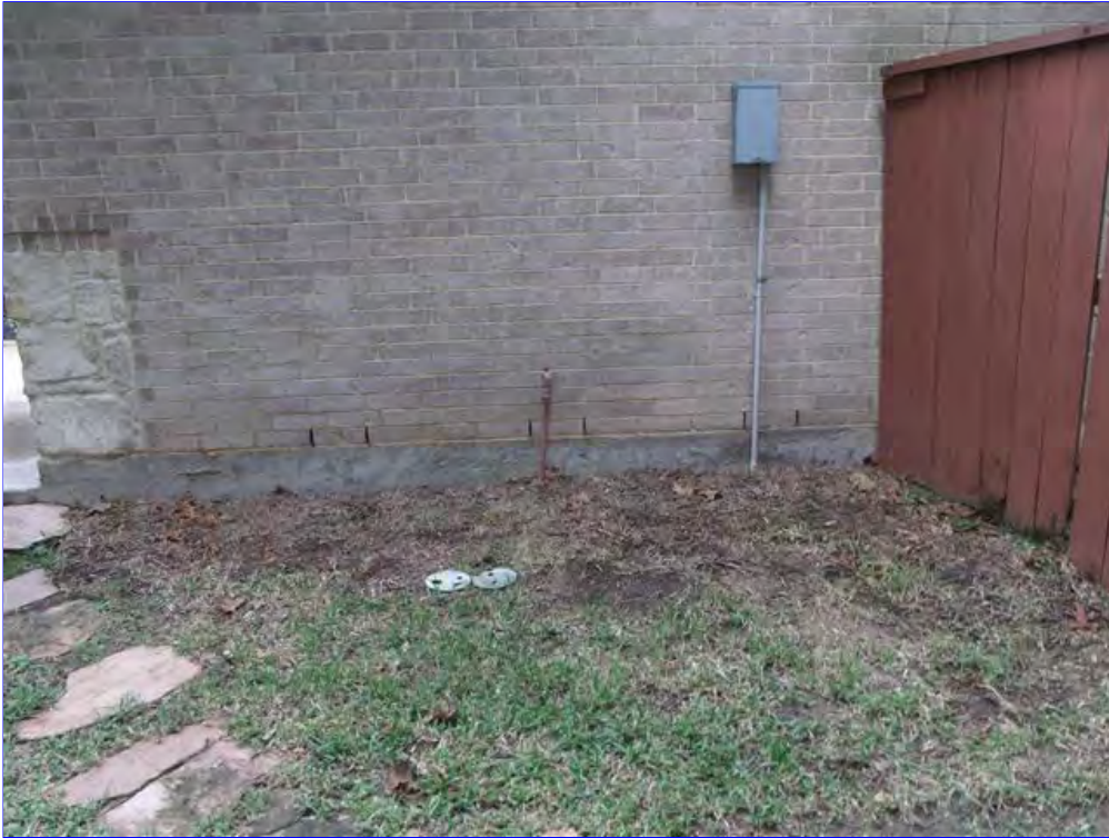
A. Item 13(Picture) Recommend having a six inch slope in ten feet away from the foundation.
