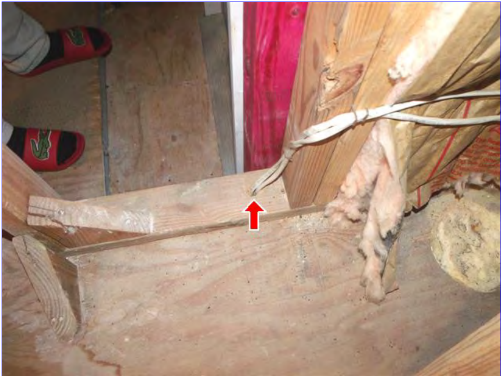
C. Item 13(Picture) Recommend sealing all penetrations
