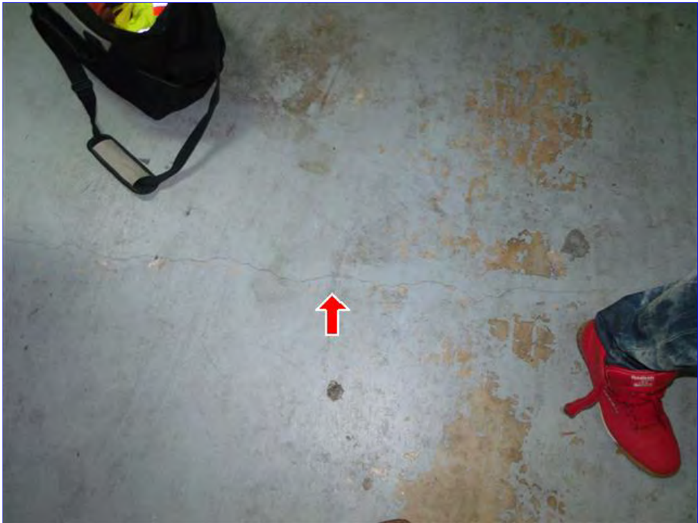
A. Item 21(Picture) Shrinkage crack on the garage floor recommend sealing with epoxy.
