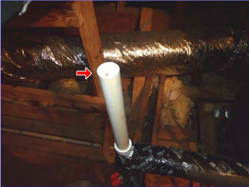
A. Item 11(Picture) Condensate line needs to be capped.
