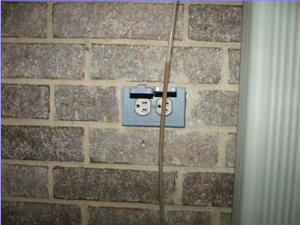
B. Item 11(Picture) outdoor electrical outlets to be GFCI.and prefer to have a water proof cover not water resistant.
