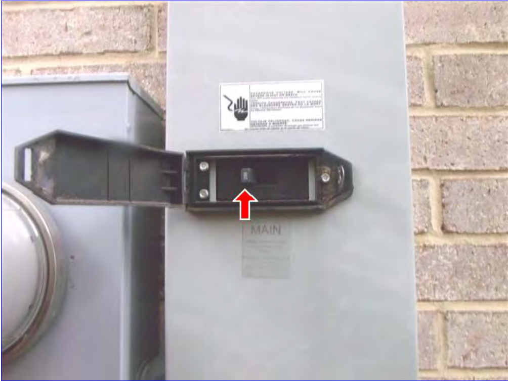
A. Item 1(Picture) Main electrical disconnect located on the right side of the house. 200 AMP power supply
