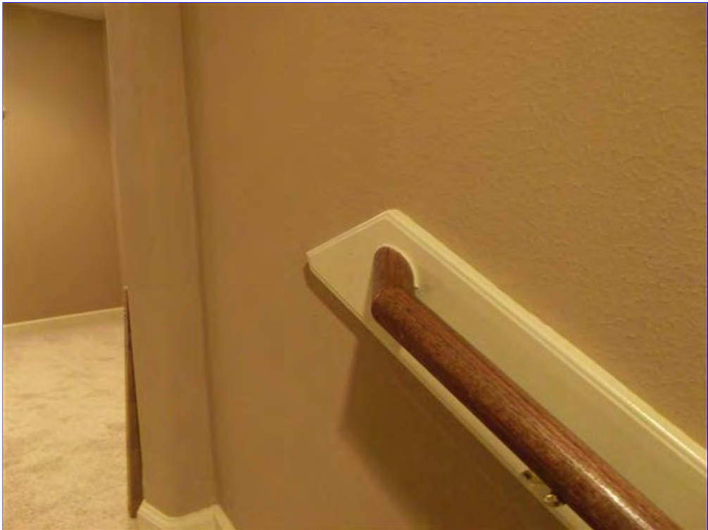
H. Item 1(Picture) Handrails need to extend past the landing.
