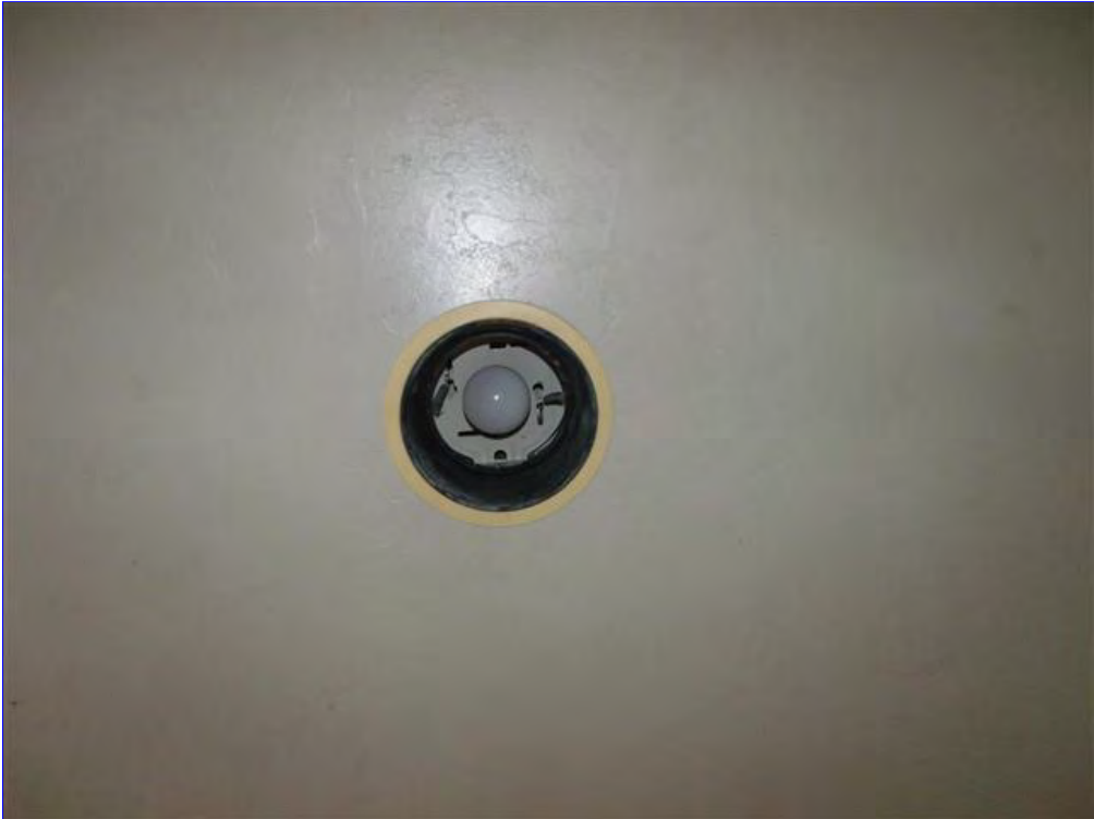
B. Item 5(Picture) Face plate for light fixture need to be installed located under the garage.
