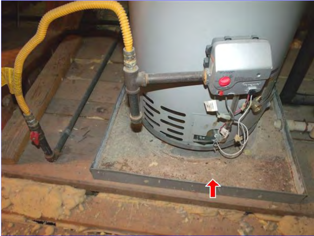
C. Item 4(Picture) Surface rusting in the drainage pan.
