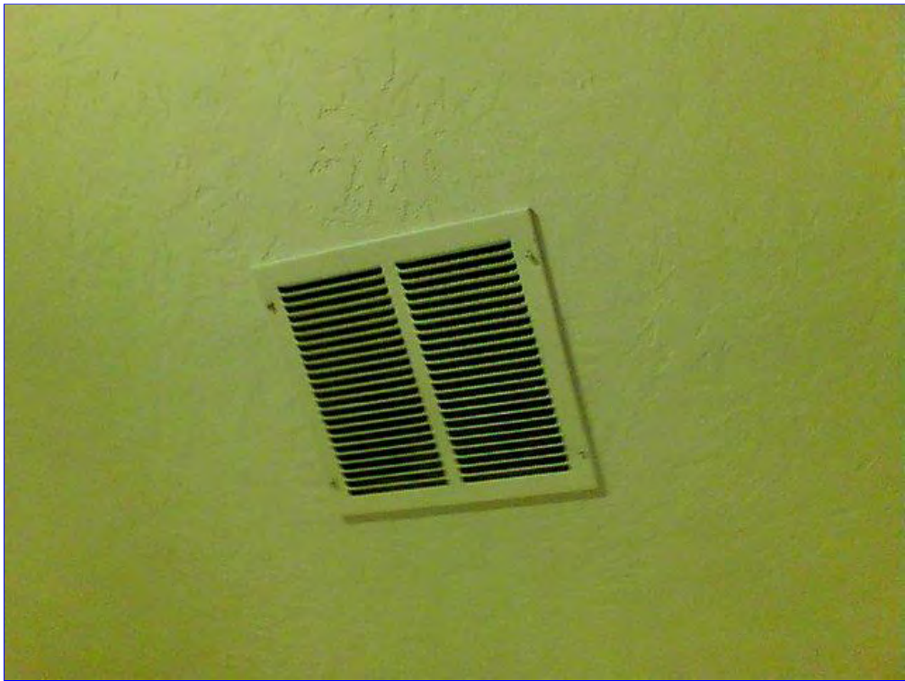
A. Item 6(Picture) Return air make sure to remove filters from inside since you have a media filter in attic that you cahange out every 4-6 months. Much better system having media filters we recommend germicidal lights as well.
