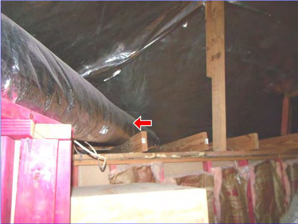
C. Item 24(Picture) Ducts need to be properly strapped.
