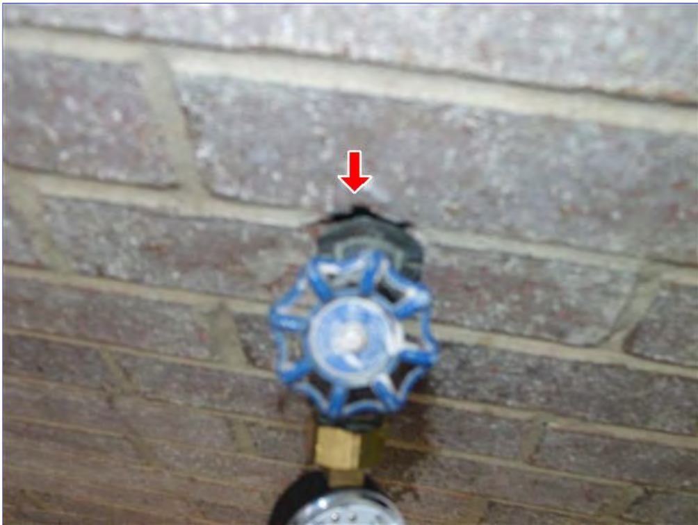
A. Item 12(Picture) Recommend caulking around fixtures.
