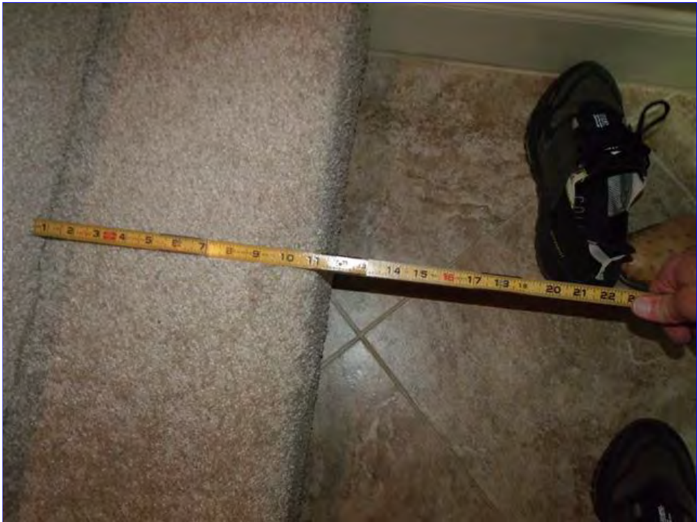
H. Item 5(Picture) Treads are deficient. Tread depth should be eleven inches with no nosing.
