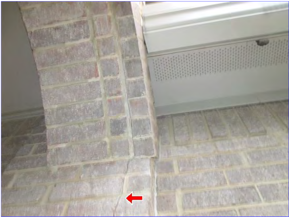
D. Item 12(Picture) Crack under the archway.
