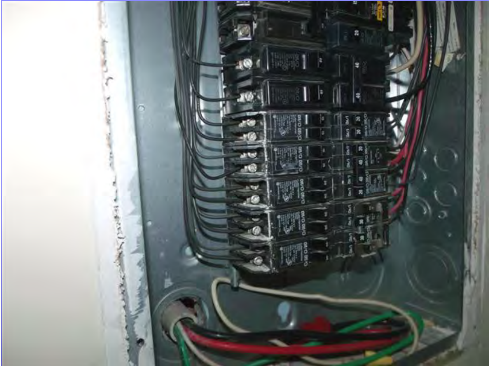
B. Item 1(Picture) Copper branch circuits.
