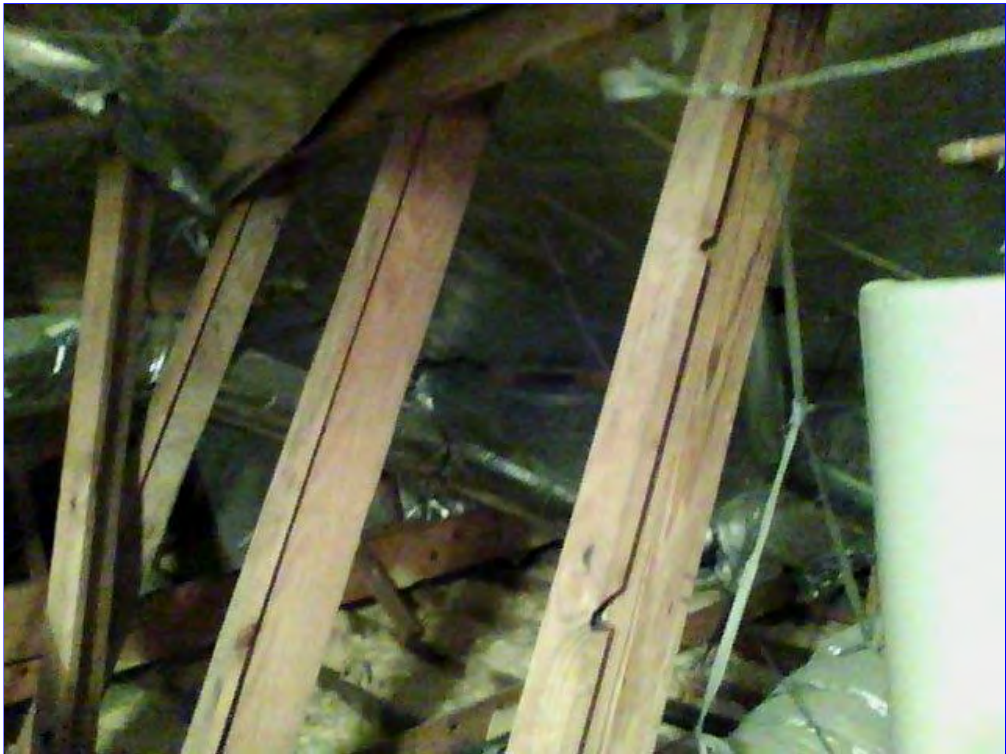
C. Item 7(Picture) Attic appears braced properly yet not all areas can be seen due to the second radiant barrier covering areas of attic.
