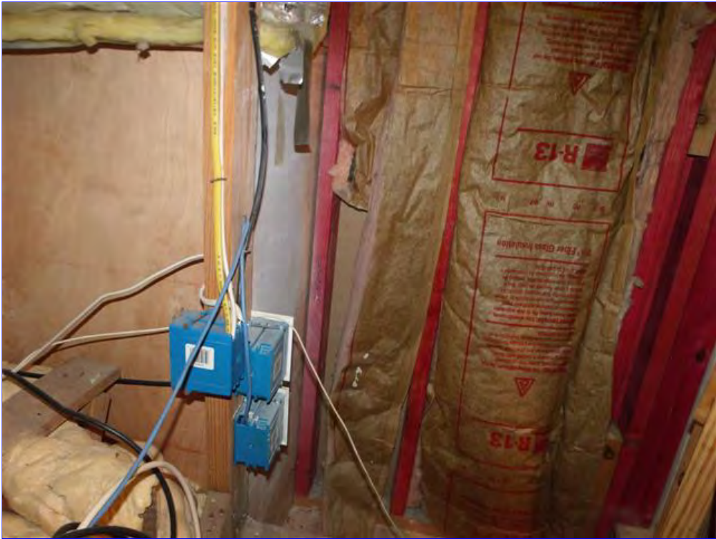
C. Item 12(Picture) Missing insulation voids in wall areas in attic after all that over kill in foam.
