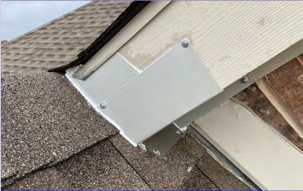
C. Item 11(Picture) Example of rodent flashing.
