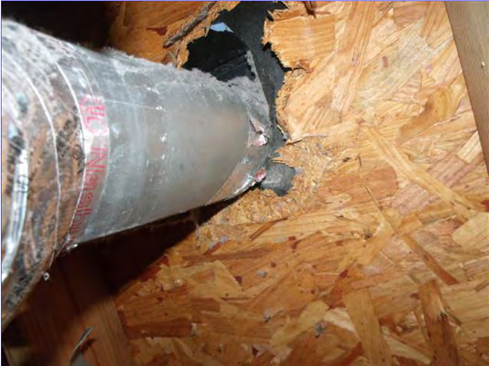
B. Item 5(Picture) IRC requires a one inch clearance for B vents.
