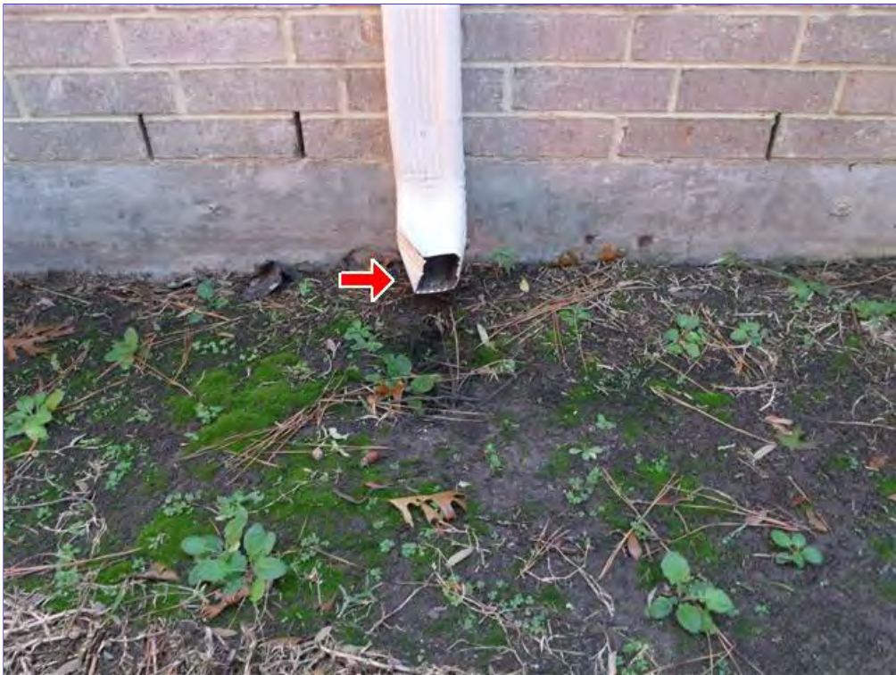
B. Item 10(Picture) Damaged downspout. Water is ponding below downspout. Recommend all downspouts discharge water a minimum five feet away from the foundation to prevent damage to the foundation.
