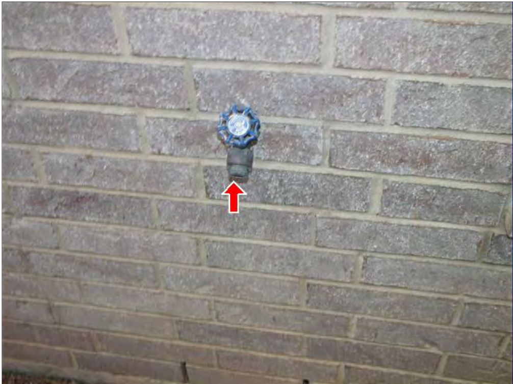
A. Item 9(Picture) Anti-siphon devices installed on outdoor plumbing fixtures.
