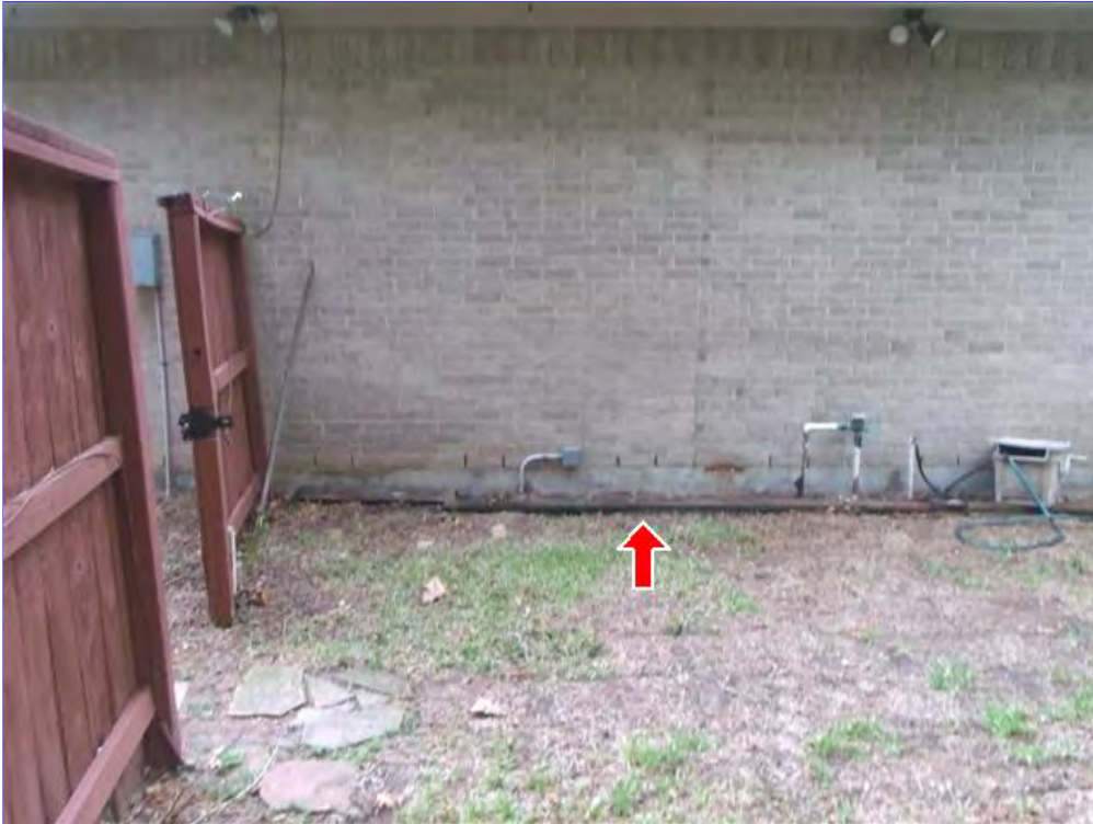
A. Item 8(Picture) Recommend clearing the wood away from the house. This is conducive to wood destroying insects (WDI) and wood destroying organisms (WDO).
