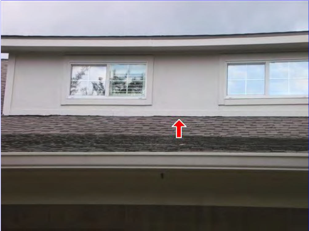
C. Item 2(Picture) Buckled flashing. In need in repair.
