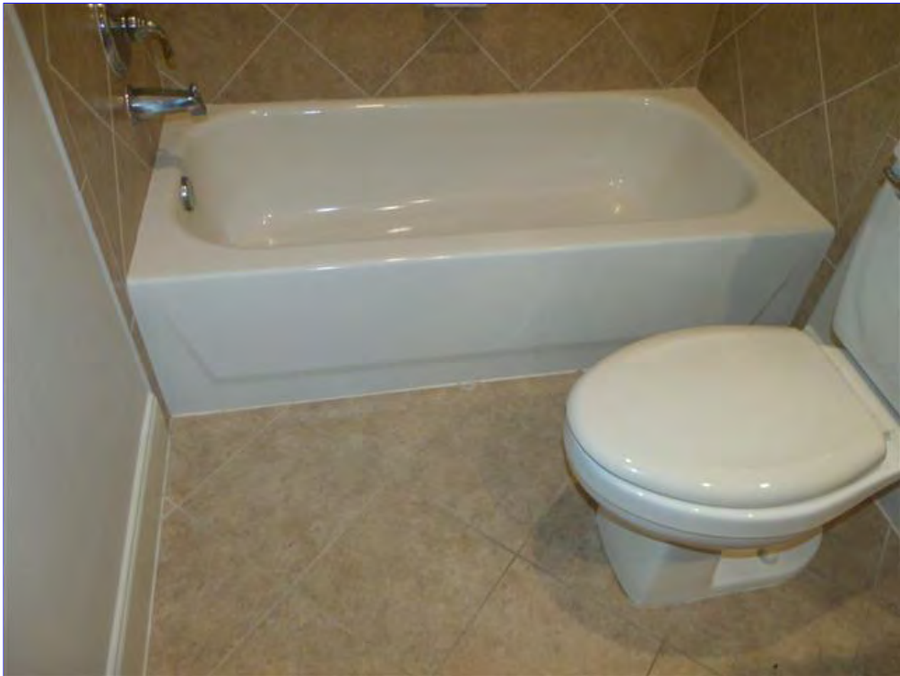
A. Item 11(Picture) No access panel is provided for the bathtub.
