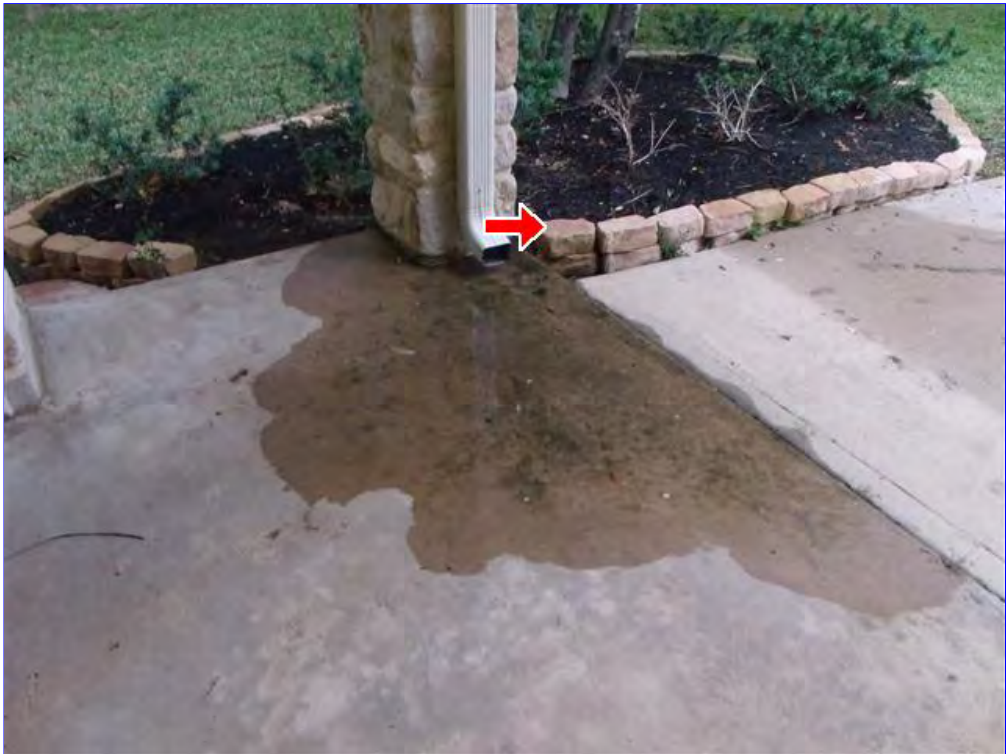
B. Item 1(Picture) Downspouts should drain water a minimum five feet away from the foundation. Turn the downspout towards the grass or add tubing to keep excessive water away from garage and driveway
