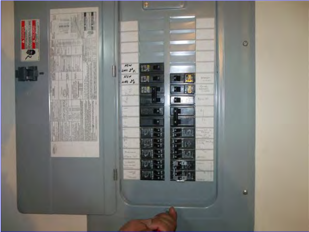
A. Item 2(Picture) Electrical panel clearly labeled.
