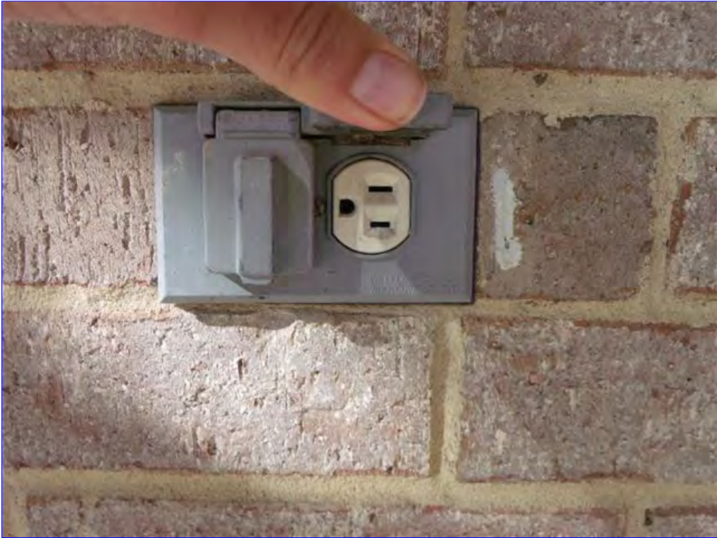
B. Item 9(Picture) IRC requires outdoor receptacles to be GFCI rated.
