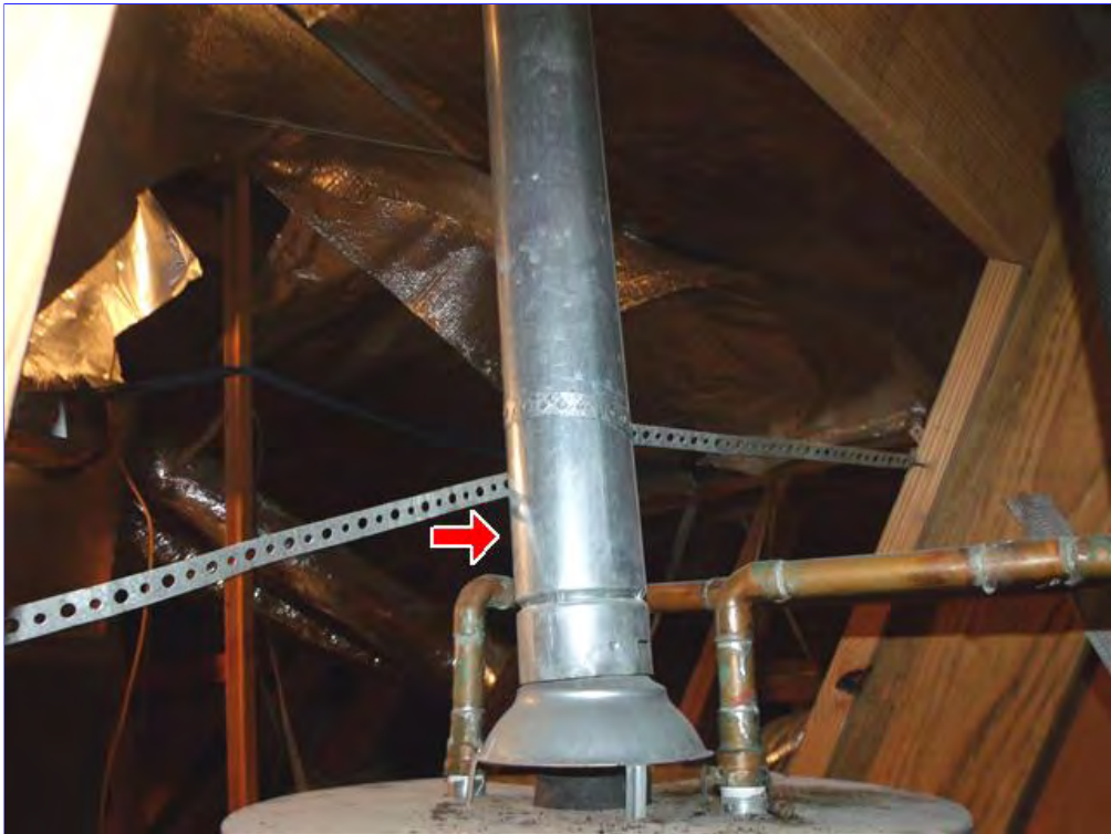
C. Item 1(Picture) Flue for the water heater should be a double walled B vent.
