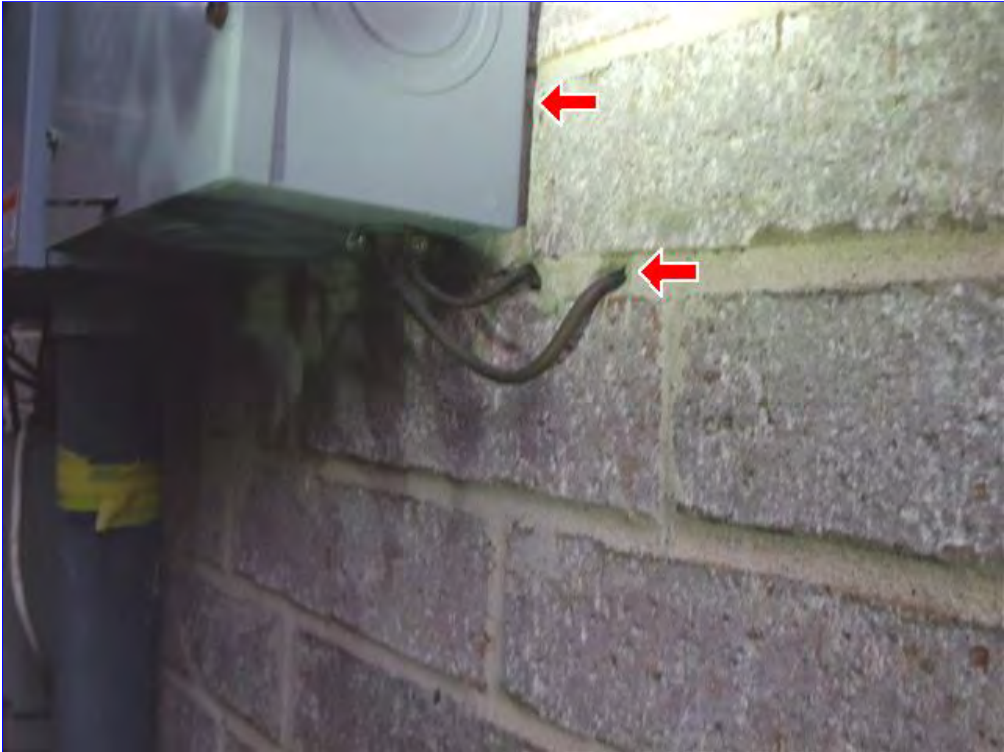
A. Item 7(Picture) Penetrations into the house need to be caulked. Electrical panel needs to be caulked to prevent water intrusion.
