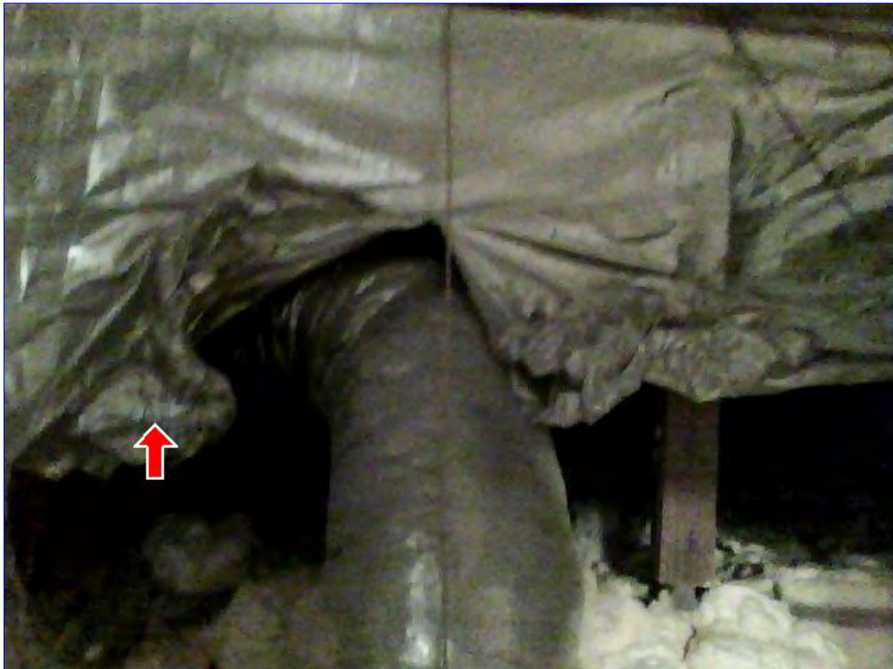
C. Item 1(Picture) Double radiant barrier installed.
