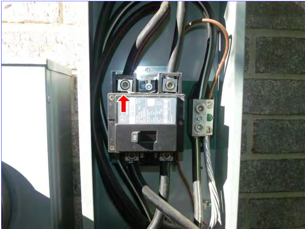
A. Item 9(Picture) Recommend capping service conductor lugs and anti-oxidant paste on aluminum conductors.
