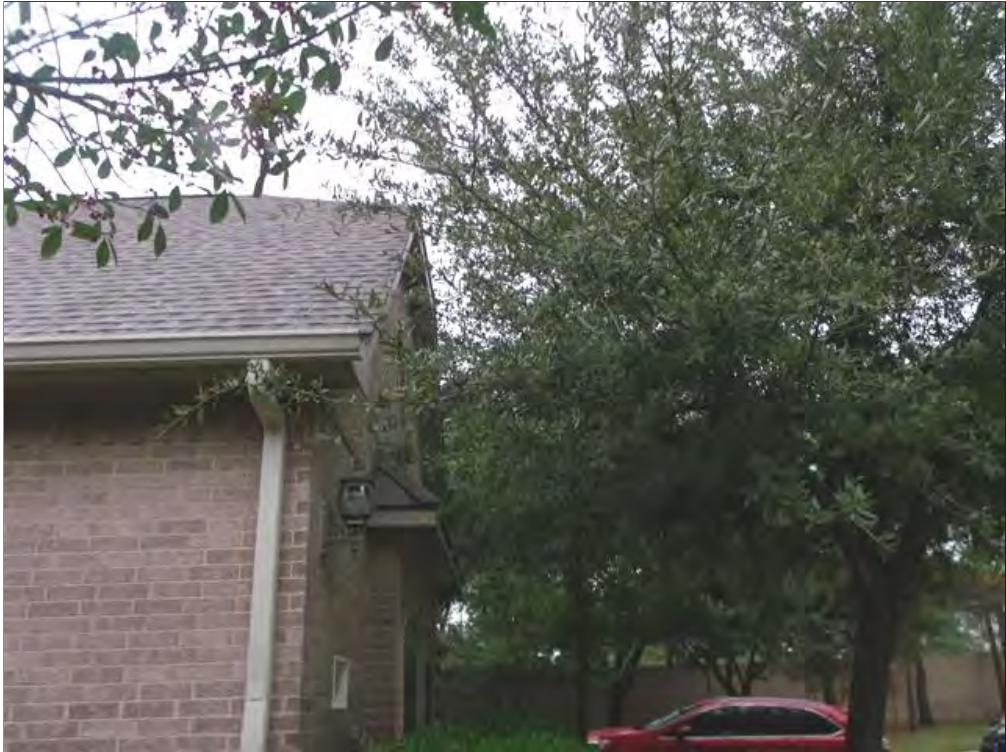
D. Item 1(Picture) Recommend cutting back vegetation. Rodents climb to roof areas and carpenter ants as well can access so make sure to cut back over hangs plus they case damage to shingles siding and gutters
