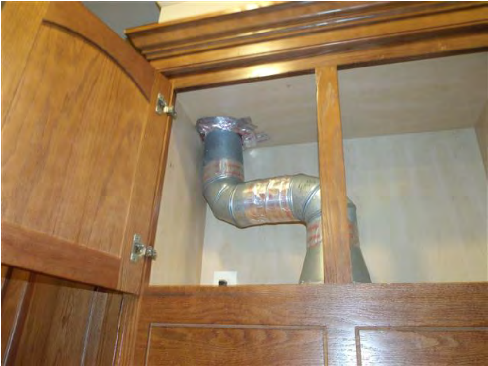
C. Item 2(Picture) Recomend adding a heat shield at top of vent and cabinet
