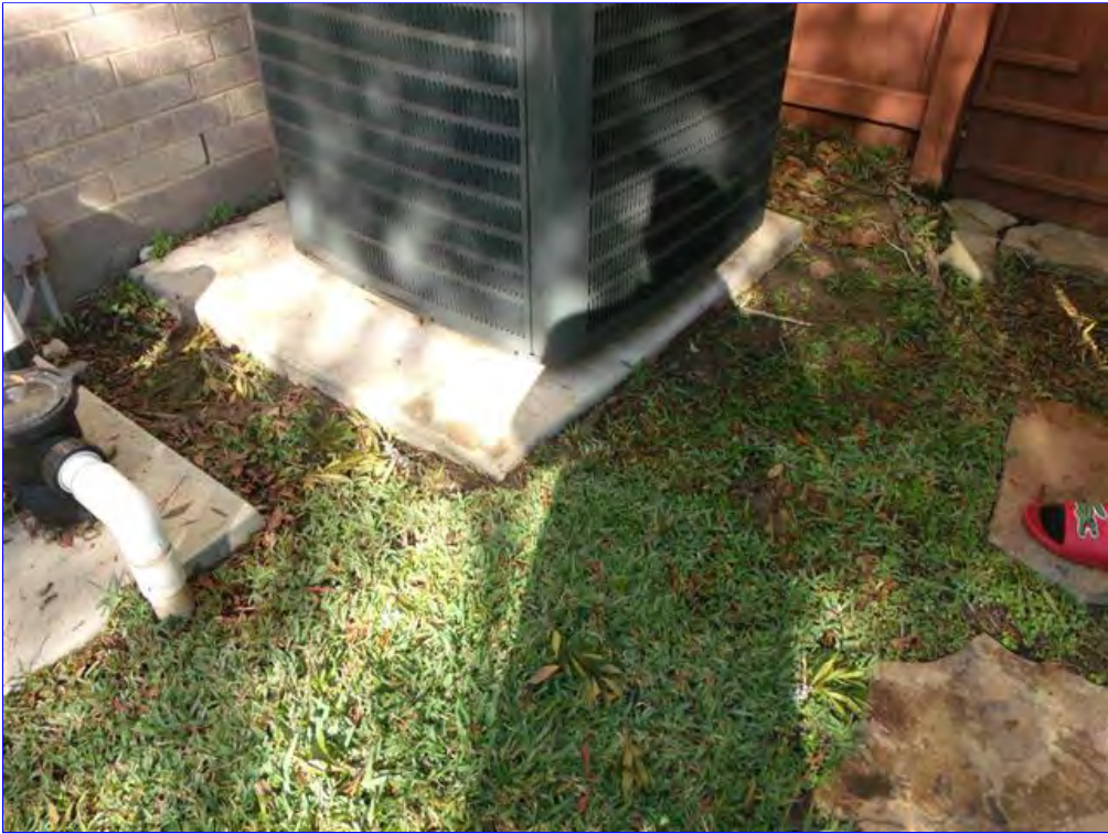
A. Item 14(Picture) A.C. unit should be three inches above grade.
