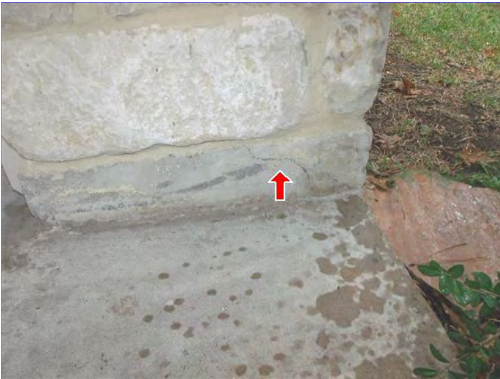
A. Item 6(Picture) Crack. Recommend sealing to prevent water intrusion to prevent damage to the masonry.
