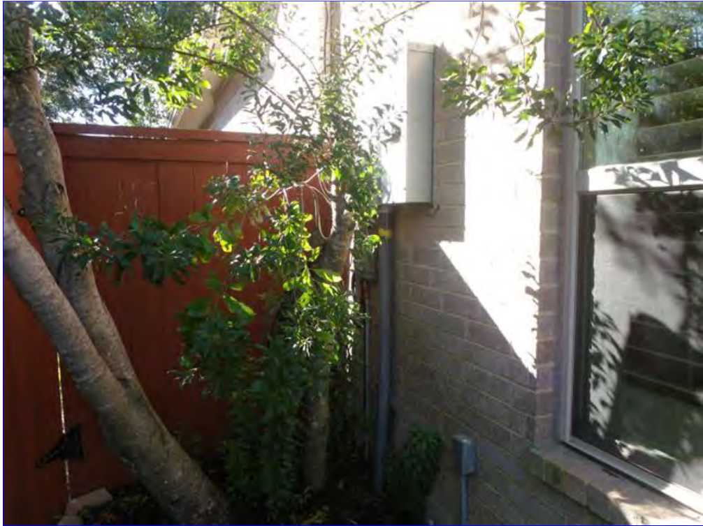
A. Item 10(Picture) Deficient. Electrical panel is obstructed.
