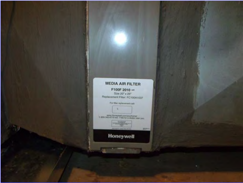
A. Item 12(Picture) Media filter provided for whole house filtration system.
