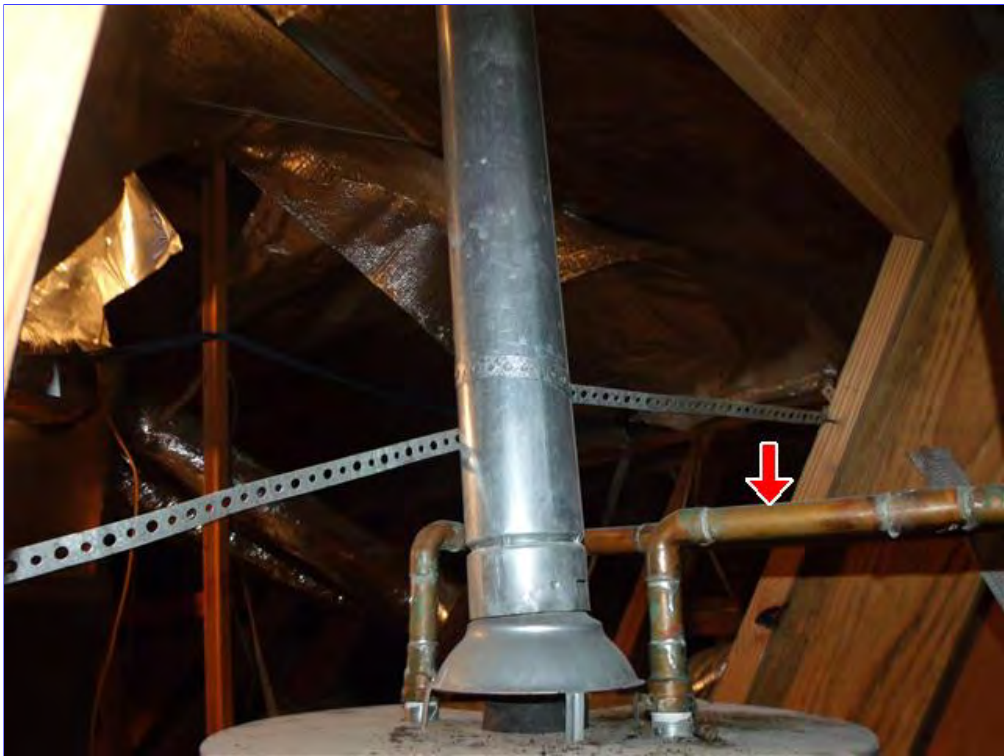
C. Item 2(Picture) Recommend insulation copper tubing starting six inches above water heater.
