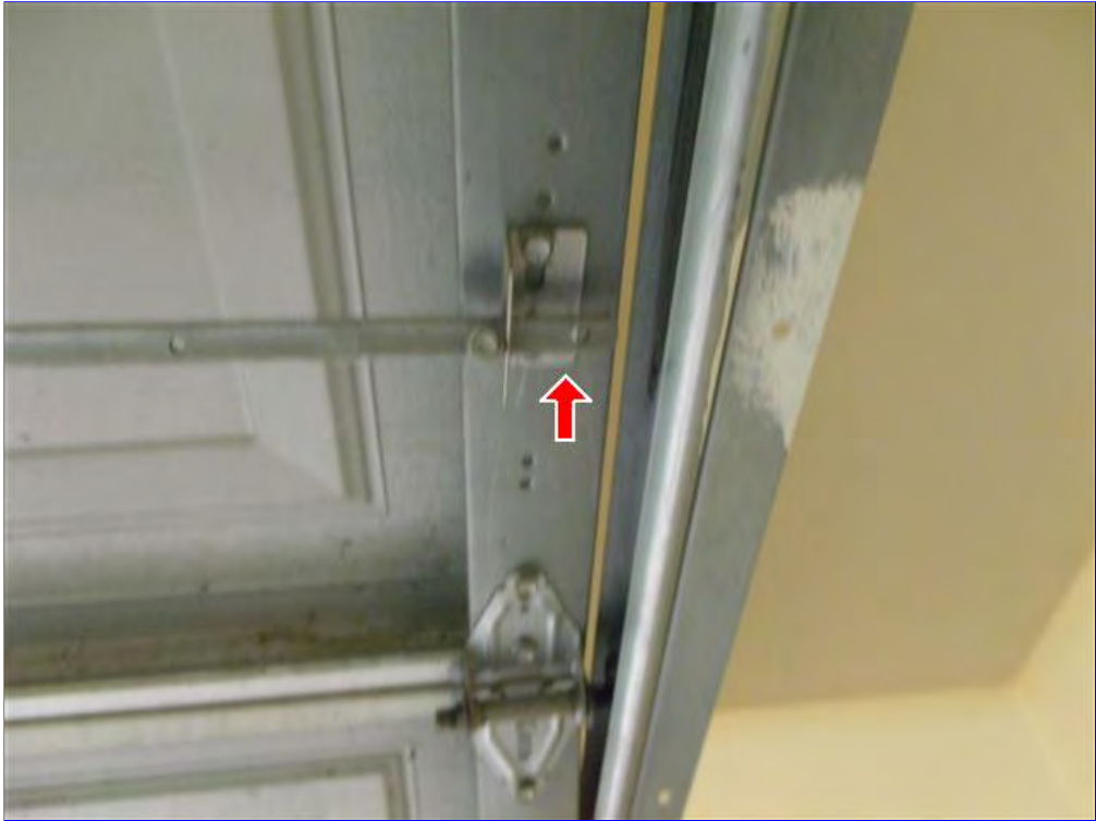
H. Item 2(Picture) Recommend disabling garage door lock.
