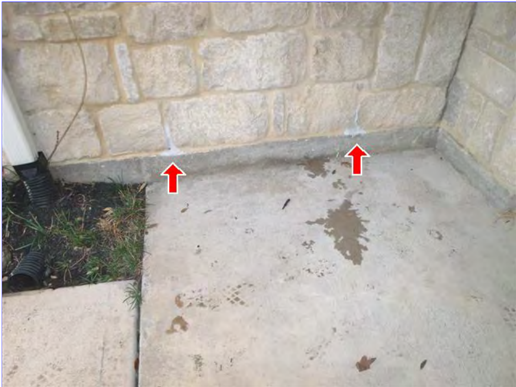
D. Item 15(Picture) Weep holes should not be sealed. Recommend repair.
